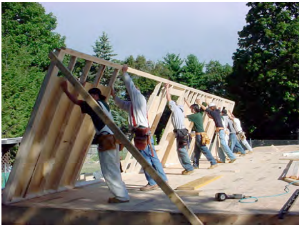
Keefe Tech students work together to frame the house.
