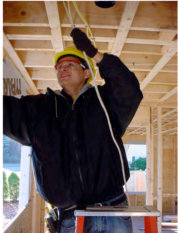
Keefe Tech senior Marone Freitas works on some wiring.
